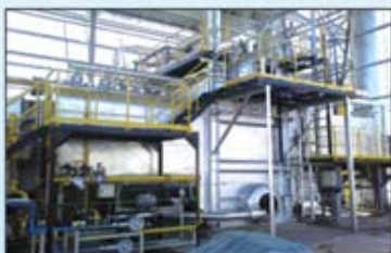
Waste Heat Boiler Model WH23SSEOG equipped with Post Combustion System
